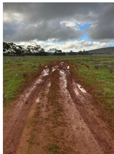
Bypass track which is now worse than the actual track.
