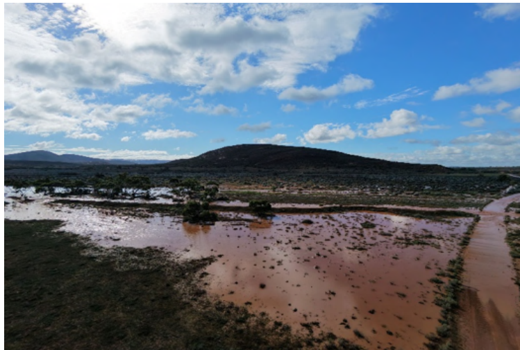
Floodwaters over track near the Shearing Shed.
